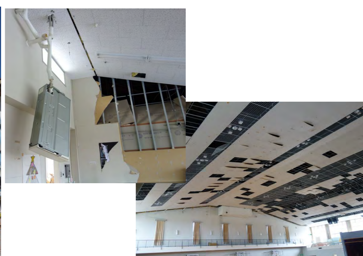
Non-structural damages
