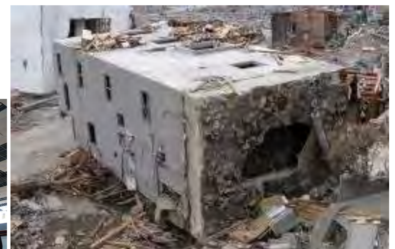
Building flushed away by tsunami
