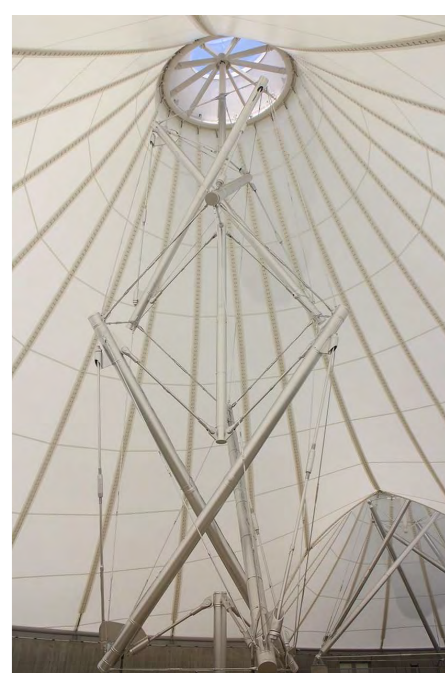
Construction of tensegrity structures
