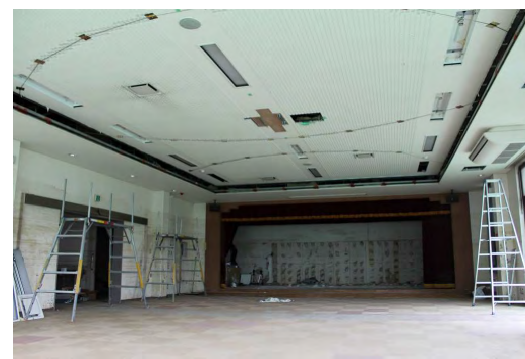
Ceiling reinforcement with cables
