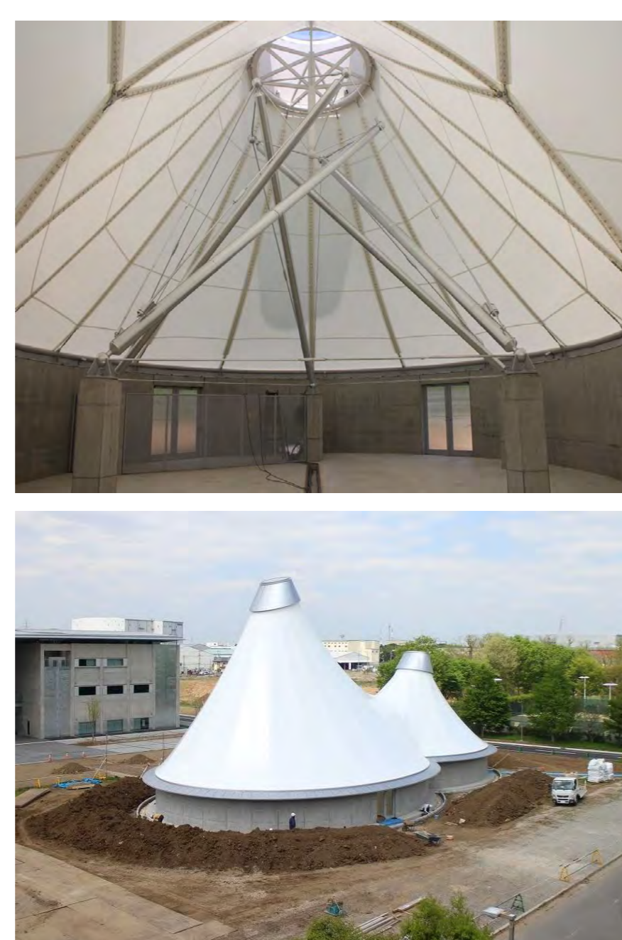
Construction of tensegrity structures
