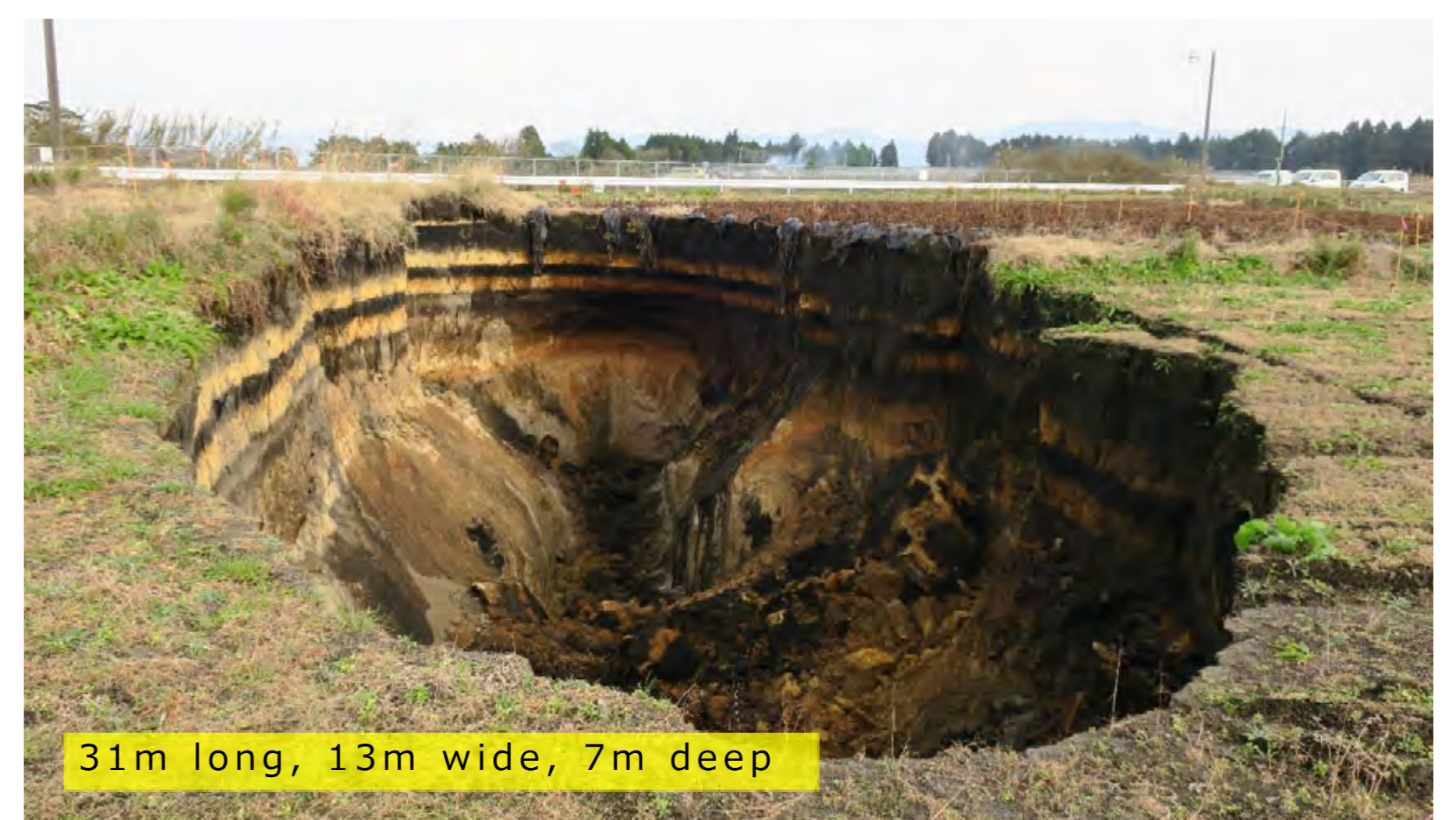
Sinkhole caused by internal erosion in volcanic "Shirasu" layer in Miyakonojo, Miyazaki (Sept. 2016)
