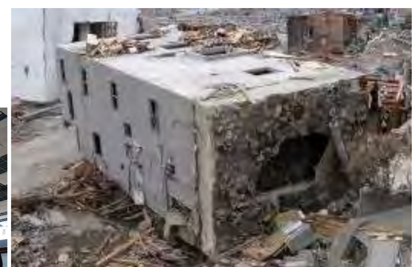
Building flushed away by tsunami
